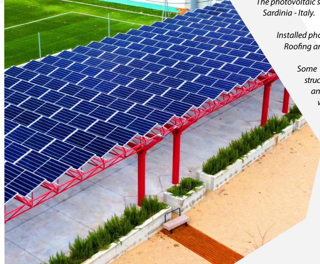
Some of the great advantages of Omnia grid structures lie in their low weight, around 18kg/m<sup>2</sup>, and the great rigidity of the connections, which allows to assemble the structures on the ground and to lift the whole body using a crane. Assembly does not require any special expertise.
